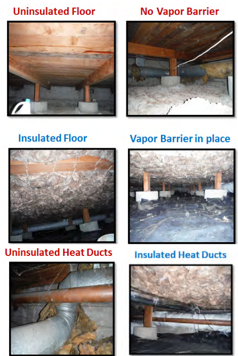
Energy Services Before & After Weatherization
